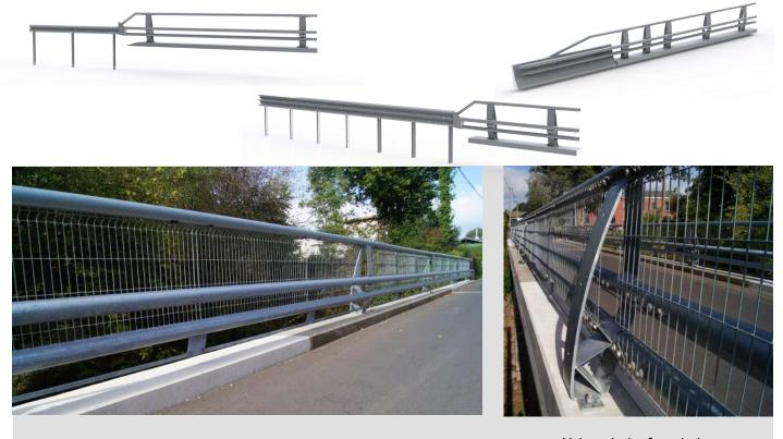
Fuse system allows the reuse of anchors after an impact
