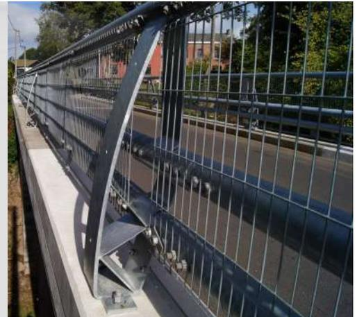
*Fuse system allows the reuse of anchors after an impact*
